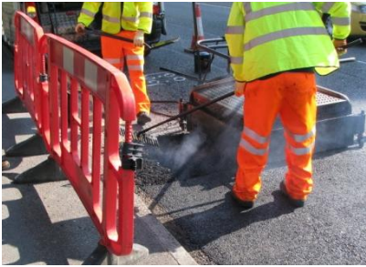
Pavement & road repairs
