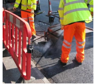
Pavement & road repairs
