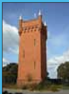
Water Tower Seafield Road
