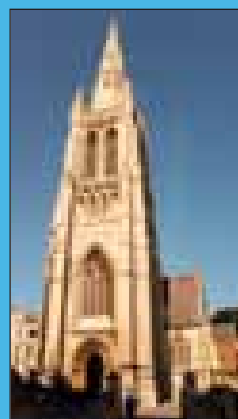
St Peter's Church Hinton Road
