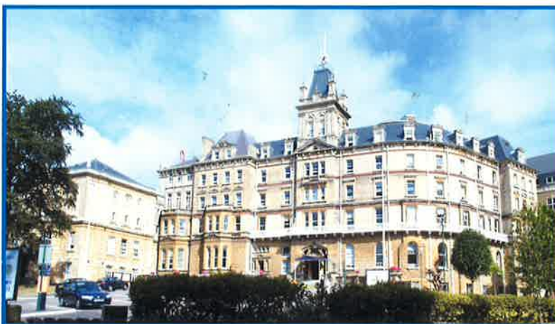
Bournemouth Town Hall, Bourne Avenue.
