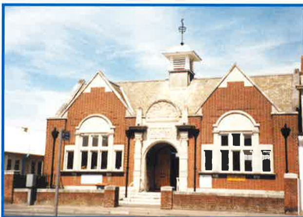
Springbourne Public Library, 293 Holdenhurst Road.
