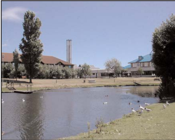
Bournemouth Hospital Example of SUDS pond
